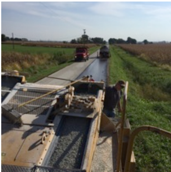
Corning Road gets resurfaced
