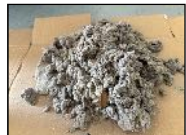
This was submitted to us by a Beecher resident who recently had their dryer vent cleaned! This pile filled over 1/2 of a GROCERY BAG!!
